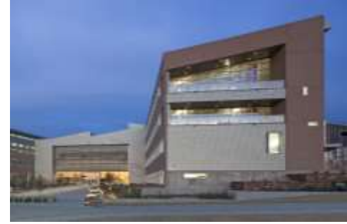
Large Office Facilities
